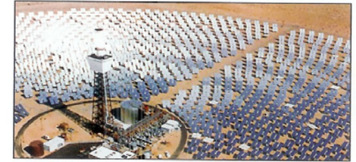
Solar 2 power tower in Barstow, California. The plant uses a combination of 60% sodium nitrate and 40% potassium nitrate as a working fluid and heat storage medium.
